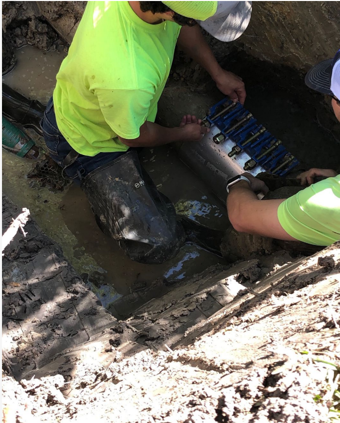
Water Main Repair
