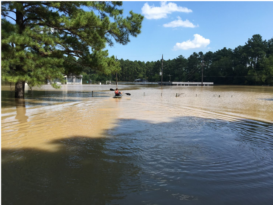
WWTP after Hurricane Harvey
