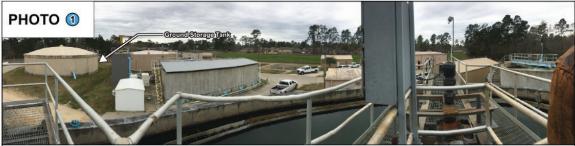
PHOTO 1 Surface Water Treatment Plant Problem: Surface Water Treatment Plant will not meet peak flows at ultimate buildout. Solution: Expand Surface Water Treatment Plant.
