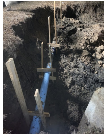
Repair to Main Line Break on Wherry Dr.
